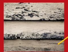
Blistering and/or peeling of outside paint. Possible cause Excessive moisture or high humidity due to poor attic ventilation
