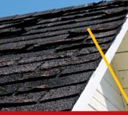
Missing, cracked, or curling shingles. Possible cause: Shingles have reached the end of their useful life.
