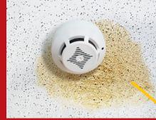
Stains on interior ceilings and walls or mold and mildew growth. Possible causes: Inadequate or faulty shingle underlayment allowing leakage, or inadequate ventilation
