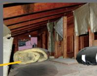
Leakage in attic after driving rain. Possible causes: Leaky or inadequate shingle underlayment; deteriorated flashing.
