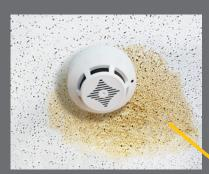
Stains on interior ceilings and Possible causes: Inadequate or faulty shingle underlayment allowing leakage, or inadequate ventilation.
